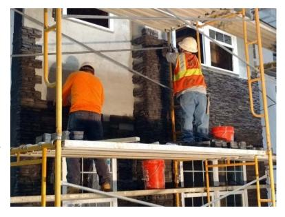
The carpentry crew time savings is related to its members' greater mastery of measuring, cutting, and attaching the cement board (from their experience working with panel products), which suggests that a carpentry crew installing PermaBase® for an adhered veneer base is the most efficient choice.
